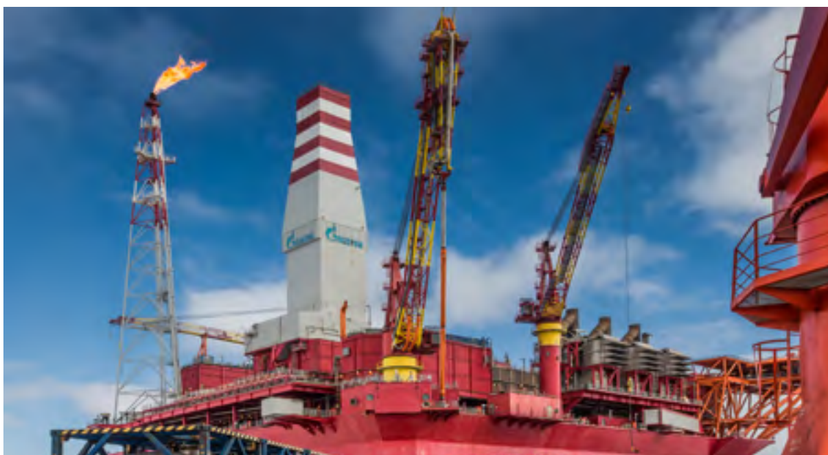
The Prirazlomnaya offshore ice-resistant oil-producing platform is seen in the Pechora Sea, Russia on May 8, 2016. Prirazlomnaya is the world's first operational Arctic rig that can process oil drilling, production and storage, as well as end product processing and loading. (Sergey Anisimov - Anadolu Agency)
